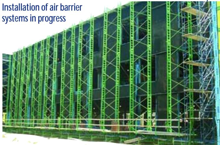
Although air/vapor barriers are intended to improve envelope performance, improper design and installation can result in water or air infiltration, condensation problems, mold growth, building deterioration and poor indoor air quality. Careful selection and placement of the air/vapor barrier materials creates an efficient system.
